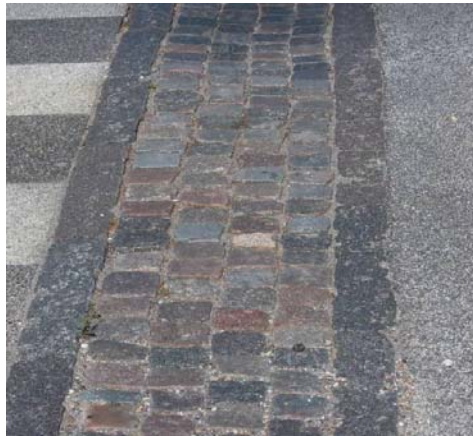
Rumble area with paving stones
