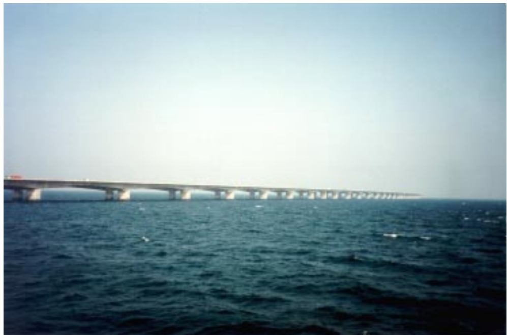
Figure 5. The 6.6 km West bridge on the Great Belt Link has two layers of epoxy primer to get assurance against blistering, 15 mm open graded asphalt concrete, 40 mm asphalt concrete (ABM) as protective course and 40 mm Stone Mastic Asphalt (SMA) as wearing course.
