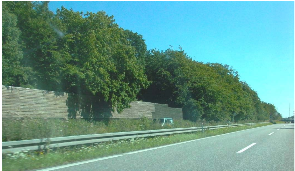
Figure 1.4. Brown wooden noise barrier adapted to the green surroundings on Highway M11 west of Roskilde, Denmark.
