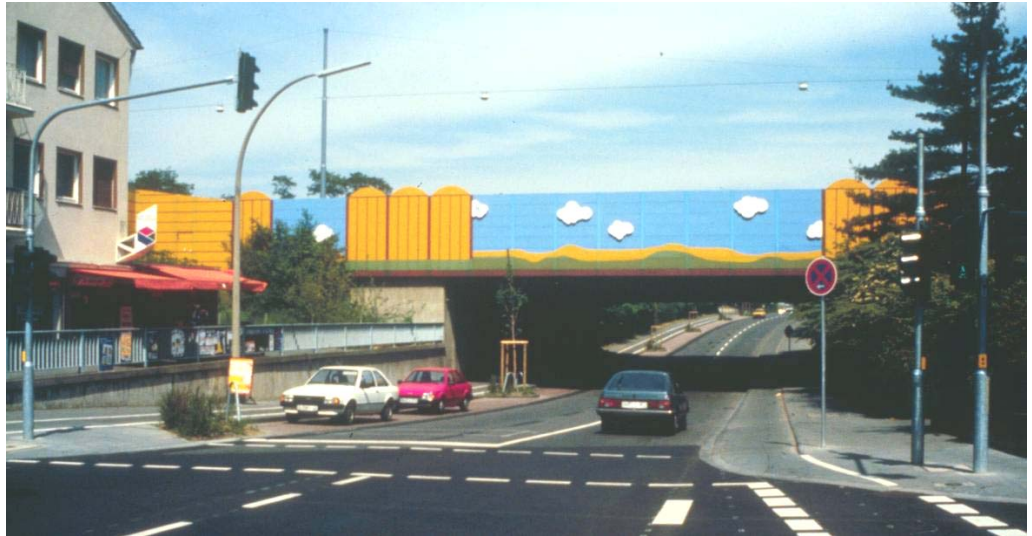
Figure 3.17. Noise barrier as a colorful urban element where Highway 555 in Germany passes on a bridge over a local road [3].
