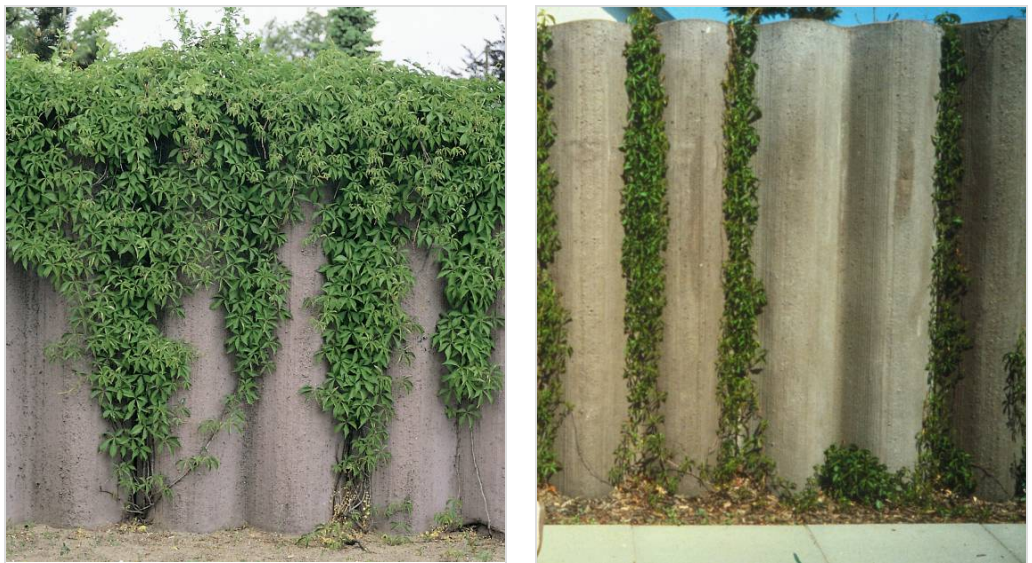
Figure 3.25. Colored concrete noise barrier made of 8 cm (3 in.) thick corrugated element with green vegetation at National Road 405 in Århus, Denmark [1, 3].
