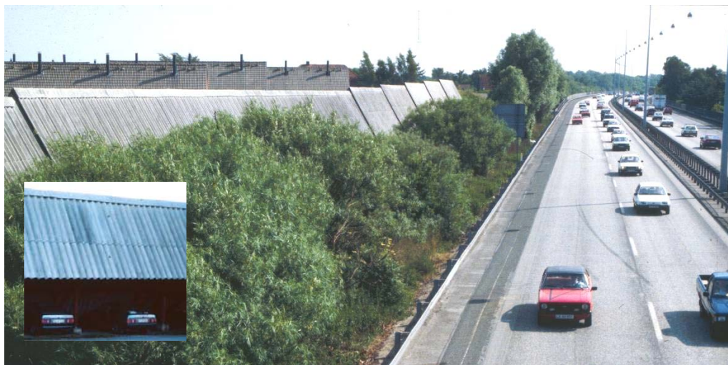
Figure 3.15. The roof of the carport construction for a residential row house area used as a high noise barrier along the M3 ring road around Copenhagen, Denmark [3].
