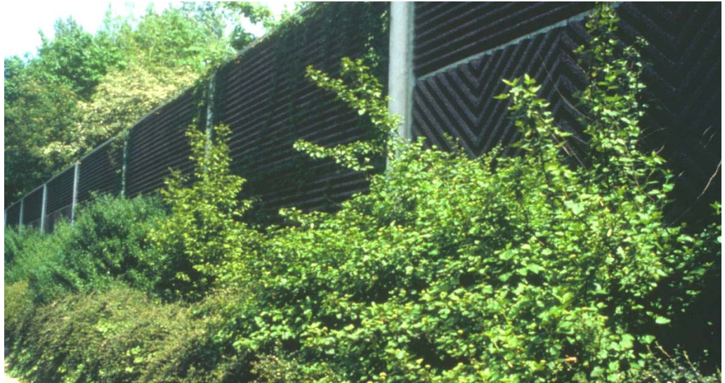
Figure 1.5. 4 m high profile brown concrete noise barriers with 1 m high plant box for vegetation along Highway A4 southeast of Cologne, Germany [3].
