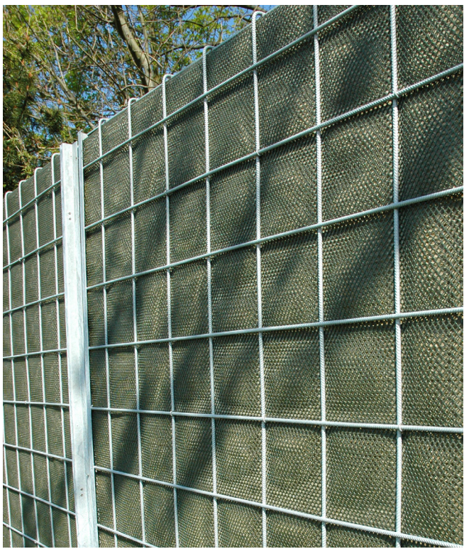
Figure 17: Noise barriers are often constructed with a surface, which is porous and therefore absorbs sound. This means that noise barriers do not reflect all the sound to the other side of the road. Often it is a porous material, usually mineral wool, on the side towards the road, covered by a perforated steel plate or planks with slits. When the cover is open in this manner, the barrier will still absorb noise.
