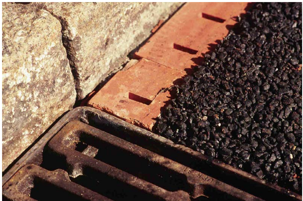
Figure 4. The drainage blocks at the roadside by the curbstones leading rainwater from the structure of the drainage pavements to the gully. The blocks have a canal inside and holes both on top and on the sidewall.
