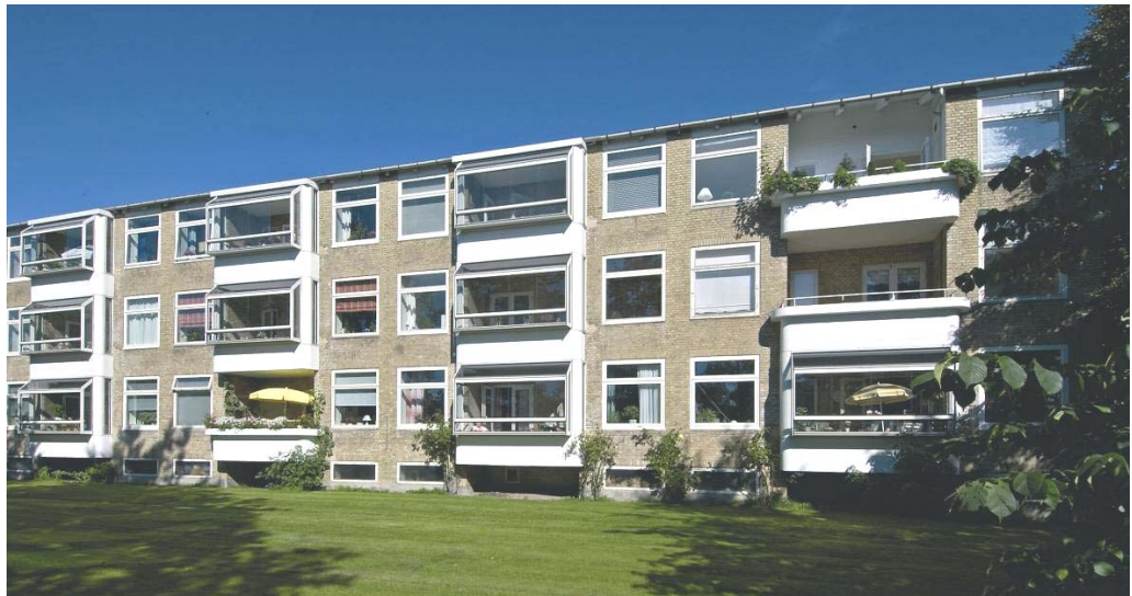
Figure 6.2. Façade insulation against noise has been carried out at dwellings along the Danish highway network and the Road Directorate has reimbursed parts of the costs.
