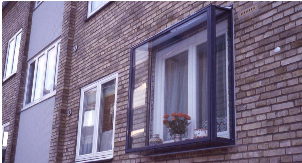
Figure 1.1. Façade insulation by applying a “glass box” in front of an existing window of bedroom or living room. Example from an apartment building in Århus, Denmark [10].
