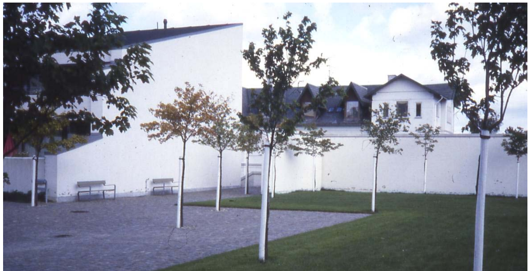
Figure 7.5. Brick noise barrier constructed as an integrated part of a new apartment building project.
