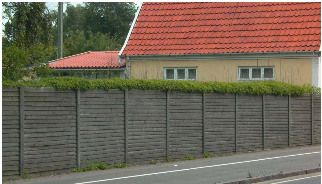
Figure 1.2. When fences at residential areas are to be renewed by the owner they can be constructed as noise barriers. This might not increase the cost significantly but the noise has to be considered when selecting design, construction and material for the new fence [10].
