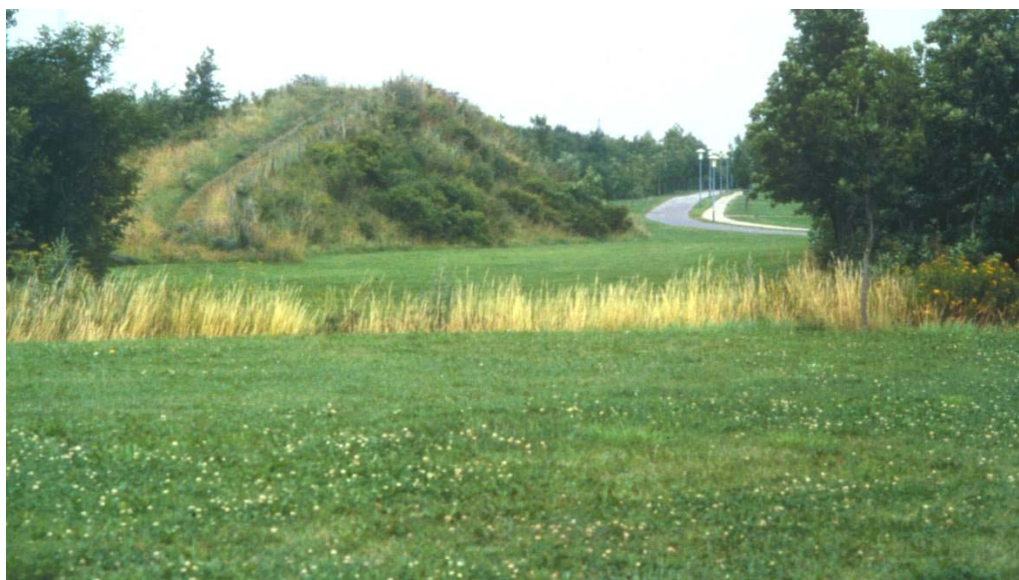
Figure 6.7. Earth embankment with a path on the top designed to fit into the urban landscape along a highway. Earth embankments can be made of surplus soil from road or housing construction projects in the region where a plan for the earth embankment is made and over a period of many years, dirt is delivered to the site before the embankment is finished. It is important to have a plan for the embankment in order to get a good final appearance in the visual environment.
