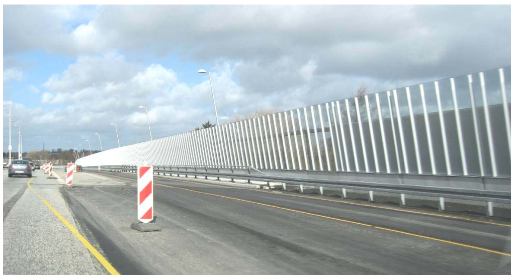
Figure 5.2. 3 to 4 m high noise barriers have been constructed along highway M3 as part of the enlargement project.
