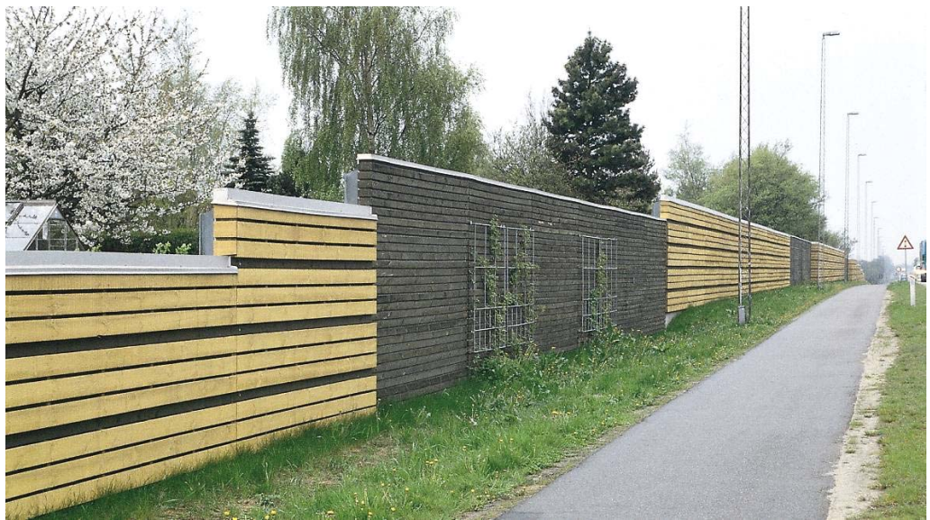
Figure 6.1. Wooden noise barrier constructed along an existing Danish highway [2].
