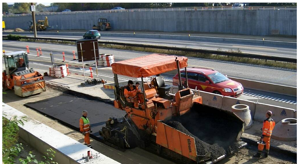
Figure 5.3. Noise reducing pavements were applied on the M3 highway.
